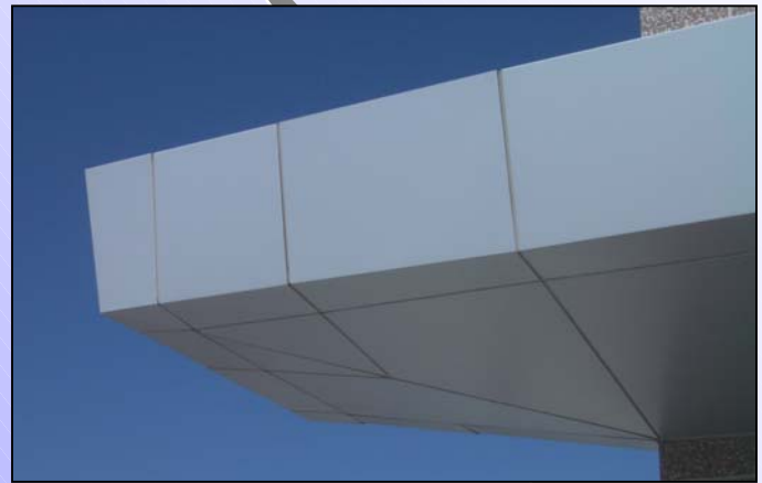
STAPLETON MEDICAL OFFICE BUILDING ROUT & RETURN ACM DENVER, CO
