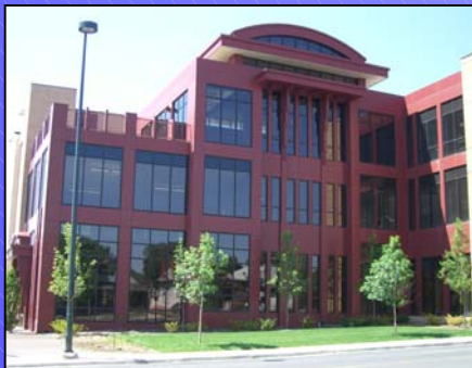
LEPRINO FOODS PANEL FABRICATION DENVER, CO
