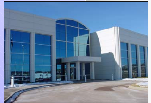
VITESSE SEMICONDUCTOR ROUT & RETURN ACM PANELS CURVED DECORATIVE CORNER PANELS COLORADO SPRINGS, CO
