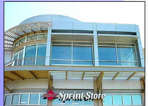
CANYON GATE PLAZA ROUT & RETURN ACM PANELS DIRECT ADHERED CURVED ACM MECHANICAL SCREEN BOULDER, CO
