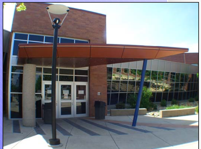
HIGHLANDS RANCH HIGH SCHOOL HIGHLANDS RANCH, CO
