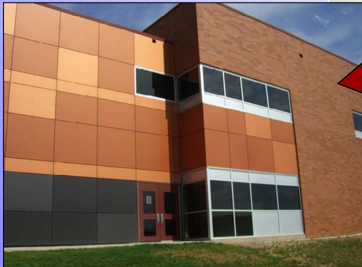
HIGHLANDS RANCH HIGH SCHOOL HIGHLANDS RANCH, CO
