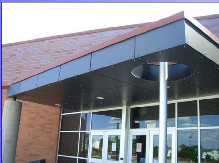
HIGHLANDS RANCH HIGH SCHOOL HIGHLANDS RANCH, CO
